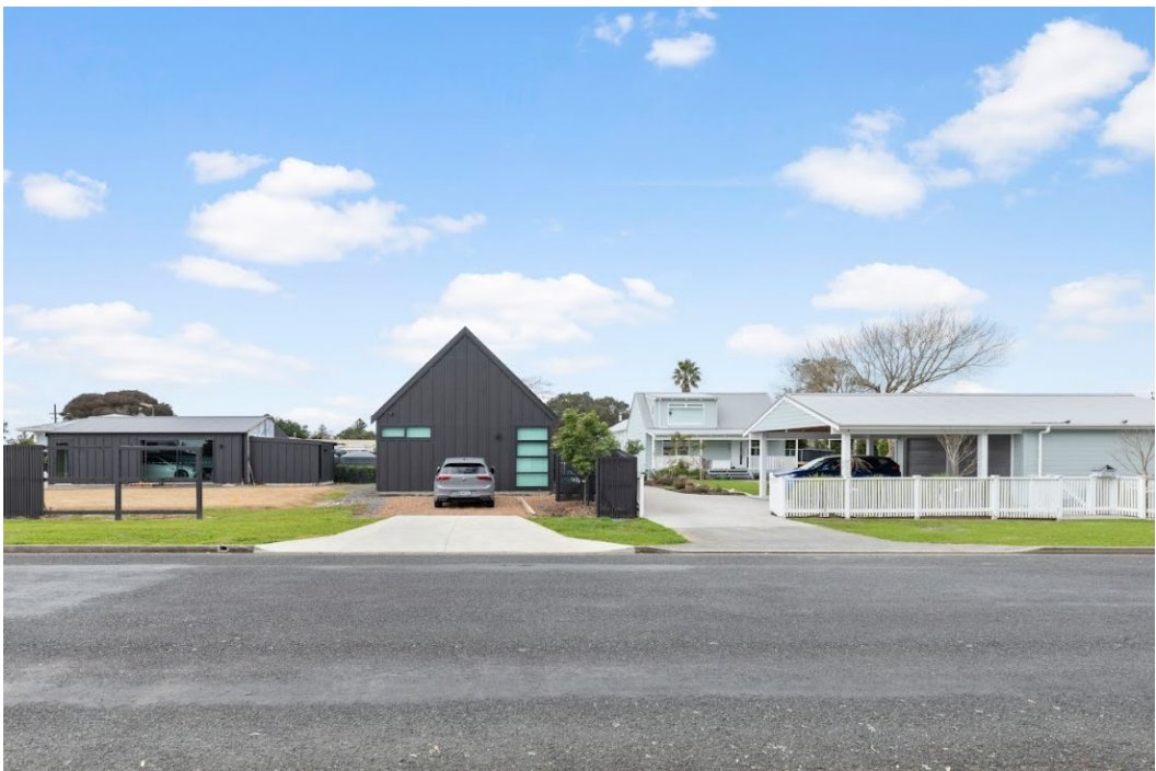
Beachlands (in progress)
